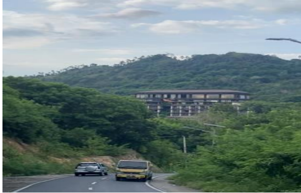
Figure 6. Taaktana Hotels Entrance Gate
